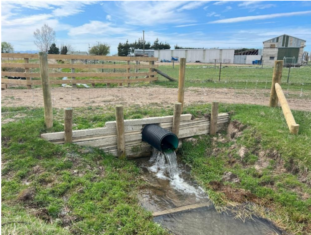
Photo 11: One of the two perched culverts installed on tributaries of the Sluice Channel sub-catchment
